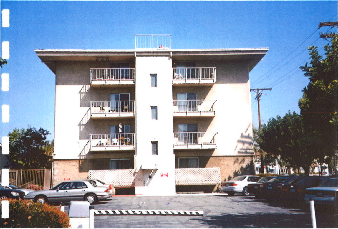
Photograph #5 Rear of Multi Story Building On Site Looking North
