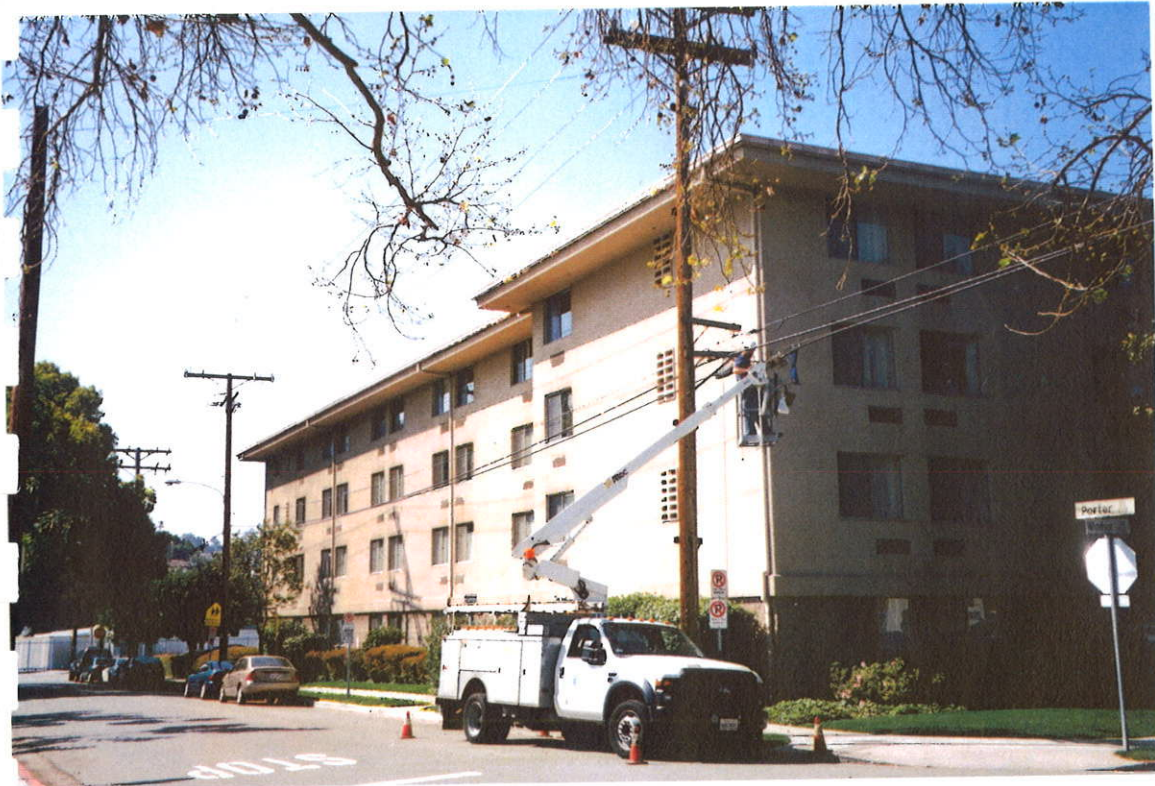
Photograph #4 Multi Story Building On Site Looking South
